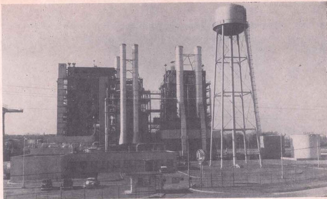
For serving Jefferson's surging industry the Louisiana Power and Light Company's Nine Mile Point Steam-Electric Generating Station located on the Mississippi River near Westwego and shown here has a capability of 319,000 kilowatts. The company also has eight major 115,000 volt substations in the parish and two others under construction, plus eleven 115,000 volt transmission lines.
