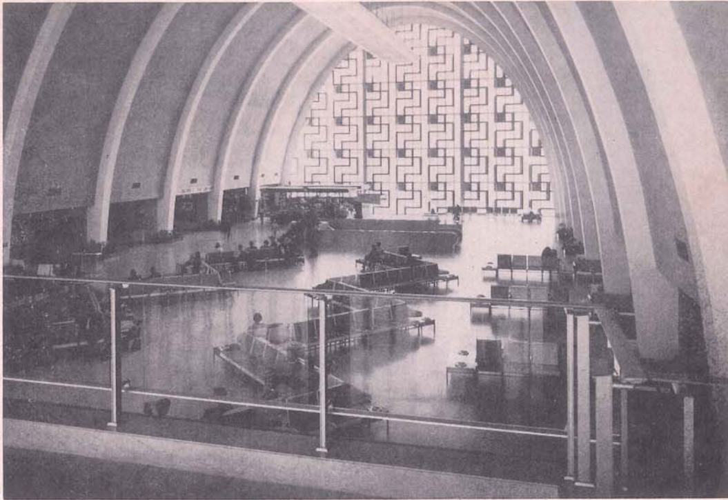
Looking down into the beautiful and spacious Main Lobby of the Moisant International Airport Terminal. It has seating room for 300, has a parabolic curved roof that rises 65 feet and high above the lobby is a 162 foot light fixture.
