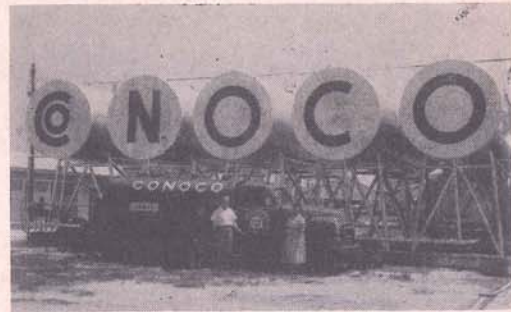
Shown above is one of the Continental Oil Company's Distribution Terminals in Jefferson Parish which supplies oil, gasoline and accessories to the service station outlets.
