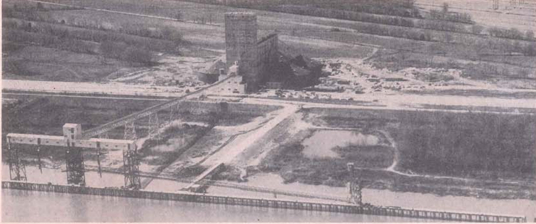
Aerial and riverfront view of the Continental Grain Company's facilities near Westwego which were completed early in 1960—showing the storage silos, the head house and conveyor belt system extending in a gallery over the river road and levee to barge unloading and ship loading facilities on the river. Continental's storage capacity can handle over 3 million bushels of grain.
