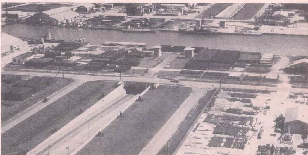
The entirely automatic vehicular tunnel which safely and swiftly carries West Bank Expressway traffic under the Harvey Canal. The opening of this tunnel drastically reduced the lost time at one of West Jefferson's most annoying traffic bottlenecks; the highway bridge on the Gretna-Westwego road that has to be raised whenever boats are moving through the Harvey Canal Locks.
