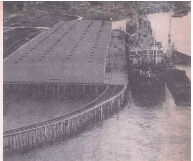
The West Bank's Perry Street Wharf which, in the few months since it has been in operation, has become one of the busiest of all wharves of the New Orleans harbor. This modern terminal can accommodate the transfer of cargo handled by two ships on several barges, 80 railroad cars and 16 trucks simultaneously.
