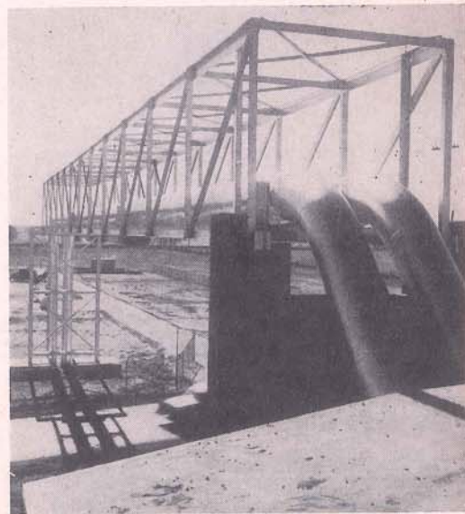
An important facet of the broad transportation story of Jefferson Parish is the pipelines which criss-cross the area to move large volumes of natural gas to markets. United Gas Pipe Line Company, transmission subsidiary of United Gas, owns and operates the lines which traverse Jefferson, and while the pipe lines emerge from underground at only scattered points, they are moving natural gas day and night. Shown here is an overhead pipeline bridge which supports two 24 inch pipe lines over a highway. The lines continue (background) to make an under water crossing of the Mississippi.
