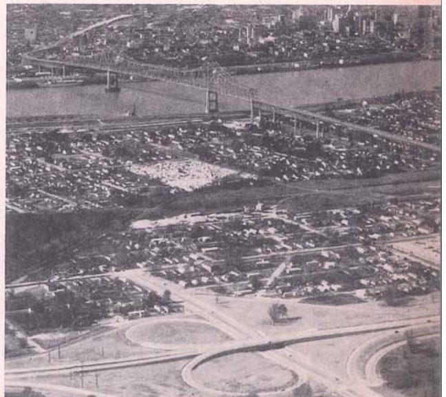
This Greater New Orleans Bridge and its system of modern approach roads serves as a vital traffic artery for expanding Jefferson Parish. The high aerial view shows the bridge from the West Bank side of the river with the New Orleans skyline in the background. Traffic on its $65 million facility is averaging more than 600,000 vehicles a month.
