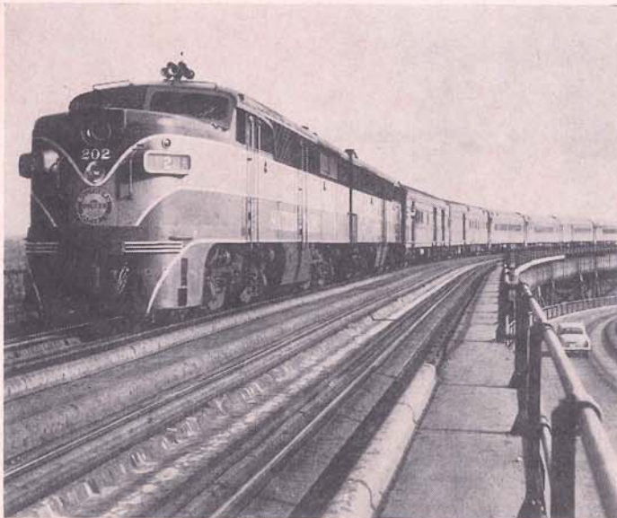
Showing the Southern Pacific's Sunset Streamliner from Los Angeles and an automobile passing each other on their separate sections of the famous 4.4 miles long Huey P. Long Bridge entirely in Jefferson Parish. When completed in 1935 it became one of the major factors in the steady march of the parish toward its present position as the most concentrated industrial area in the Deep South.
