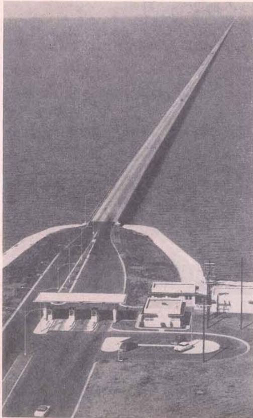
Showing the Jefferson Parish approach to the Lake Pontchartrain Causeway, the world's longest bridge spanning 24 miles of open water and four miles of approaches.
