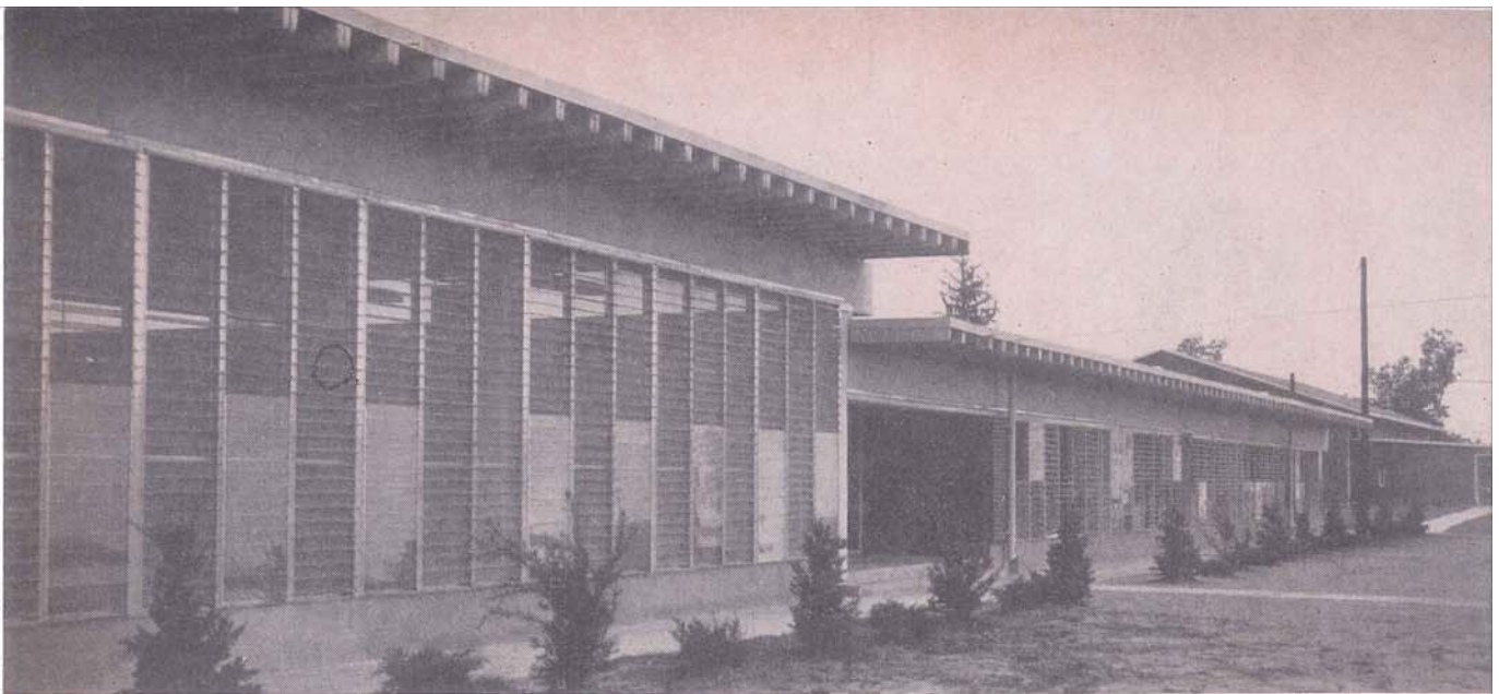
Exterior of Westgate School to which ten new classrooms and cafeteria were added for the opening of the 1959-1960 school year.
