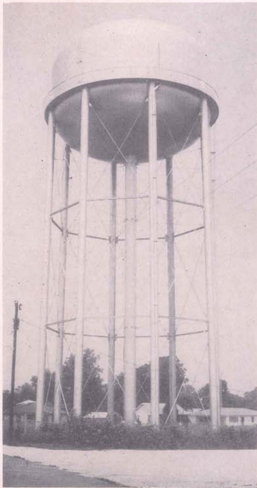
New 1/2 million gallon elevated water reservoir of Waterworks District No. 3 at 16th and Allo Streets in Marrero.
