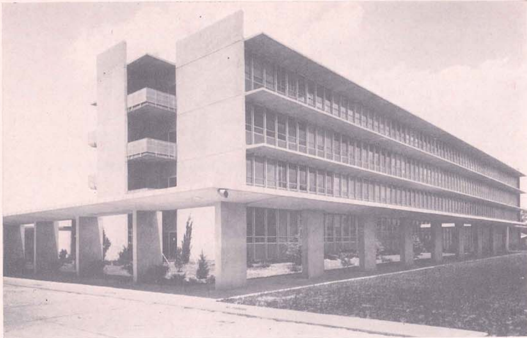
Showing the front of year-old 159-bed West Jefferson General Hospital at Marrero. Now occupying only ten of the twenty acres it acquired, the vacant area in its front provides the space for future expansion around a central quardangle.
