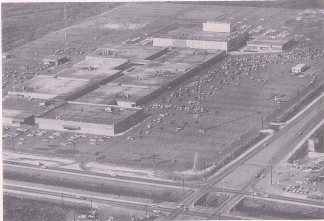
Aerial view of the East Bank's great regional Shopping center Lakeside Shopping Center, located at Veterans Highway and Causeway Boulevard. Lakeside is comprised of 36 stores under one roof, including many of the leading names in the retail industry. Lakeside offers one of the largest parking facilities in the South. Over 5000 cars can be accommodated. Each store opens on to the Mall where there is no vehicular traffic, allowing for pleasant, safe leisurely shopping.
