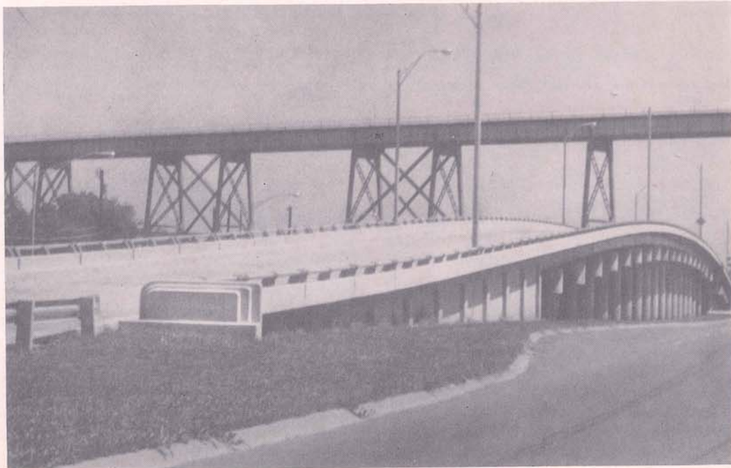
The new time and snarl-saving overpass on Jefferson Highway at the Huey P. Long Bridge which permits traffic from Harahan or Kenner to move straight through without having to maneuver the traffic circle at this point. The overpass continues a four-lane highway through Harahan to Williams Boulevard at Kenner.
