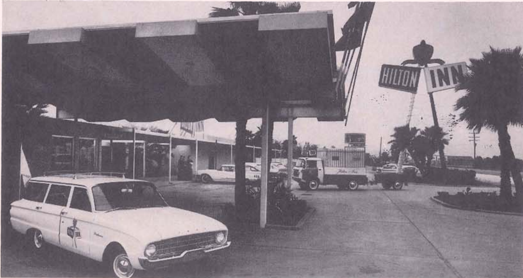
Some of the country's finest motor hotels are located in growing Jefferson Parish. The ultra modern Hilton Inn, located just across from Moisant International Airport, has 310 guest rooms in addition to complete banquet and meeting facilities. In addition to catering to air travelers, the Hilton Inn has brought a number of large conventions to Jefferson Parish for the first time.
