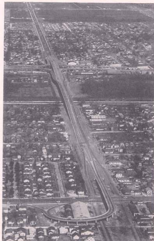
This picture of modern East Jefferson shows the Overpass System to the Lake Pontchartrain Causeway, expediting traffic throughout the East Bank.
