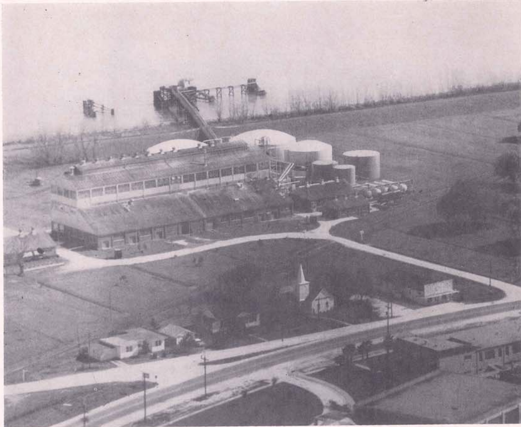
The Belle Chasse plant of Red Star Yeast and Products Company. Producing active dry yeast for baking, this plant serves domestic and international markets. The first of its kind in the country, this plant was designed to produce 100% of its production as active dry yeast. Strategically located in a molasses importation center, the plant is also in an excellent position to make export shipments to any continent through the Greater New Orleans Port. In addition, large volumes of water are available from the Mississippi River for processing and cooling.
