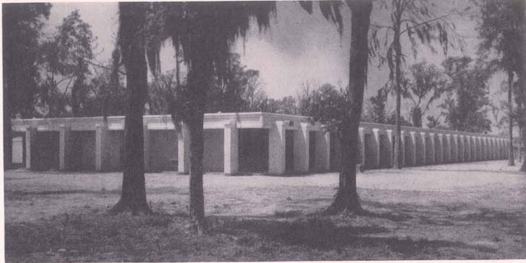
Above: The new Ralph J. Bunche Junior High School with 32 classrooms cafeteria and administration wing, now in use in the Kenner area. Below: The new Fourth Ward Elementary School of 22 classrooms, cafeteria and administration building, now in use at Marrero. Ninety-nine new teachers were added this year to meet the increased educational demands.
