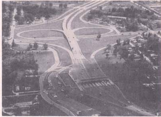
Victory Drive Interchange and Mississippi River Toll Plaza looking toward Jefferson Parish on West Bank Expressway. Bridge incline starts at lower right of picture.
