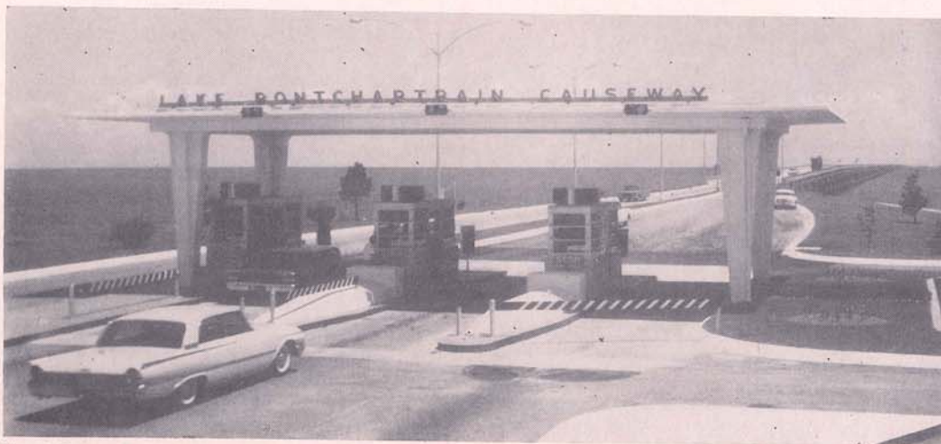
The Jefferson Parish entrance and exit to the Lake Pontchartrain Causeway, the world's longest bridge. This 24-mile long bridge, which serves the parish as a direct North-South thoroughway route, completes its sixth year of operation on August 30, 1962.
