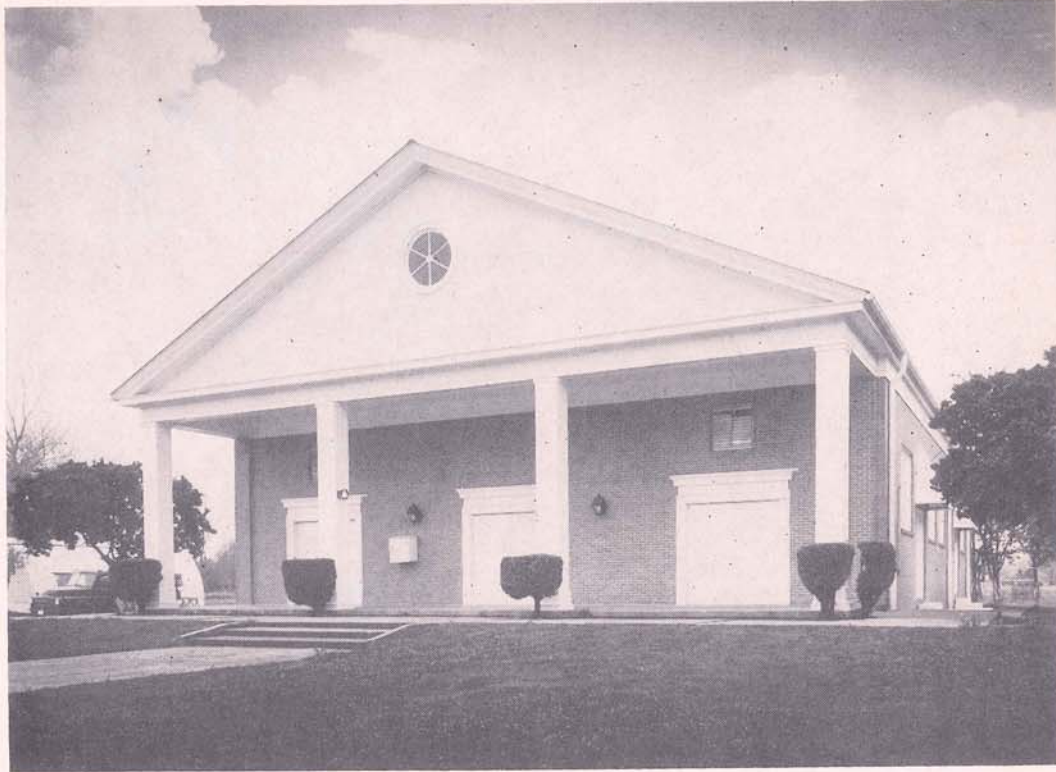
At Belle Chasse the Plaquemines Parish Community Center and Auditorium which was renovated in 1961. It is the West Bank headquarters for community affairs and the new parish-wide recreational program.
