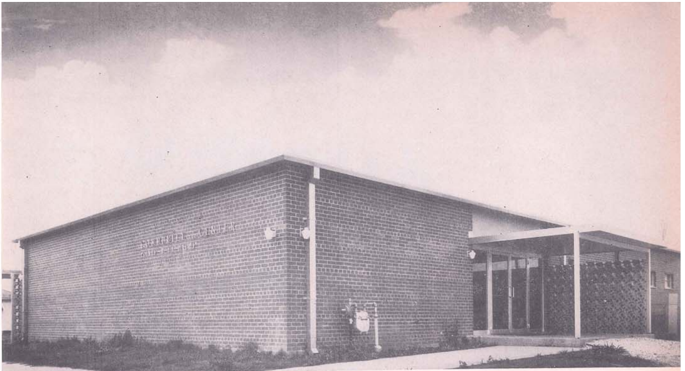
The new Community Center at Pointe a la Hache completed in 1961. This is designed for civic, social and community affairs on the East Bank and is part of the new parish-wide recreation program.
