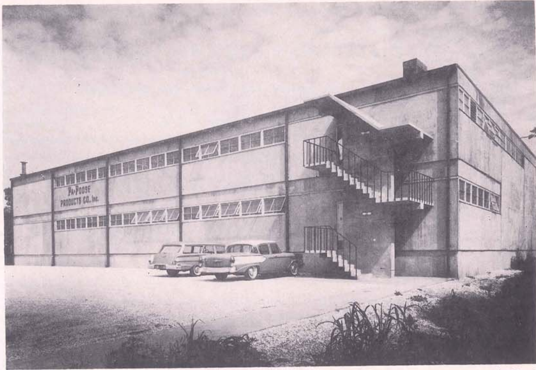
The new million dollar plant of Pa-Poose Products Company at 82 First Street in Gretna. Recently D. J. "Buddy" Olistter, General Sales Manager of the new Pa-Poose Company, signed a contract with the executive committee which holds the Little League Baseball franchise in the area to sponsor 100 teams in Jefferson Parish and New Orleans. He immediately ordered 1500 uniforms and equipment for the youngsters, age limit 10 to 12, who will form these teams. All games will be supervised by the Jefferson Parish Recreation Department with tournament play beginning June 15 until August 15 with regional playoffs, state playoffs and then to National and International Championships.
