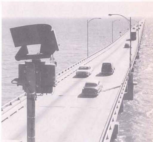
Radar installation helps safeguard motorists
