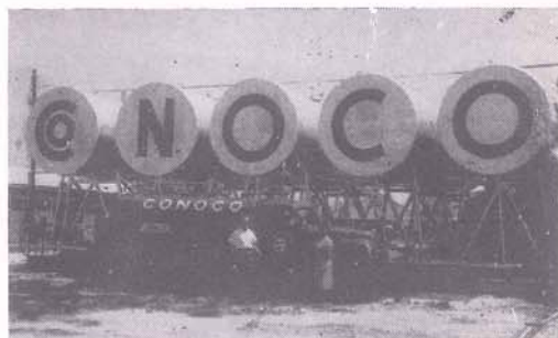
Shown above is one of the Continental Oil Company's Distribution Terminals in Jefferson Parish which supplies oil, gasoline and accessories to the service station outlets.
