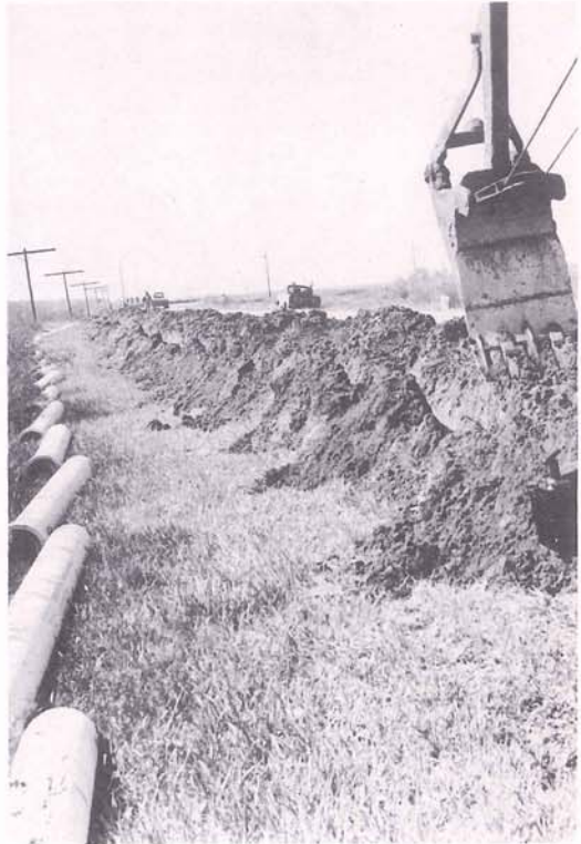
Showing construction of the Grand Isle water distribution system.
