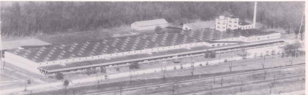
Gulf Atlantic Warehouse Co.'s Shrewsbury Industrial Center located at Labarre Road and the I. C. Railroad. This is one of Jefferson Parish's largest commercial facilities providing both general merchandise warehousing and distribution and leasing space for both commercial and light industrial tenants. The complex known as the Shrewsbury Industrial Center has a 45 acre tract of industrial land adjacent to it for future development and expansion for industries that wish to locate in growing Jefferson Parish.
