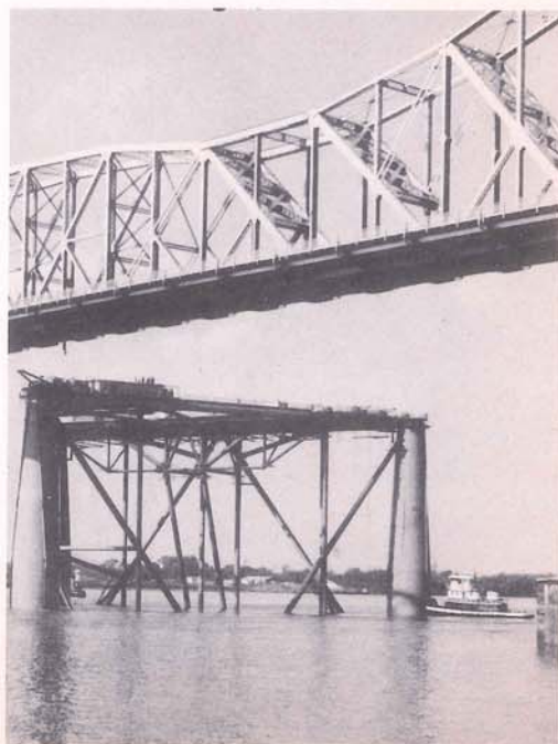
Below: The KERR-McGEE Rig 54 as it passes under the Huey P. Long Bridge on its way from Avondale Shipyards to a location in the Gulf of Mexico. This is the largest structure ever moved down the Mississippi River. Five tug boats and one push boat were used to tow it downriver. This $6½ million rig measures 206 feet from its base to the top of the workers' deck.
