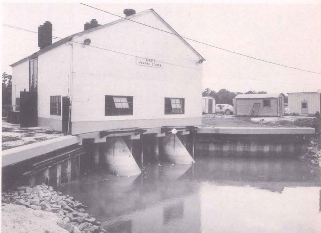
The Ames Pumping Station—recently repainted, inspected and kept at maximum efficiency—part of the West Bank Drainage Construction and Upgrading Program throughout the populated portion of the West Bank unincorporated areas.
