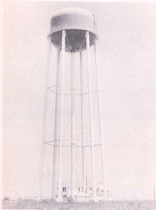
One of the water storage tanks of Grand Isle's new waterworks system that was officially turned on May 18, 1963, marking the end of cypress cisterns. It now serves Grand Isle's homes and business establishments and the Humble Oil and Refining Company Base on Grand Isle, which had barged in 21 million gallons of potable water the previous year. Grand Isle's present plentiful supply of water comes from Lafourche Parish through a pipeline that runs 18 miles to Leesville. Grand Isle is now also served with natural gas, from the Tennessee Gas Transmission Company which carries a natural gas trunk line northward across the island.
