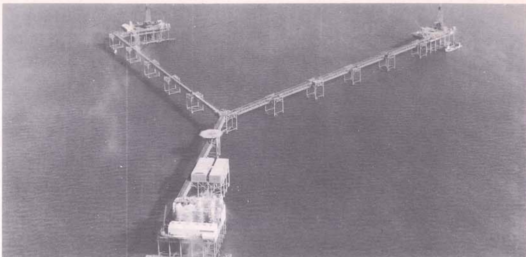
The Freeport Sulphur Company's offshore sulphur mine in the Gulf of Mexico seven miles from Grand Isle. It is the first of its kind in the world. This huge steel island—a series of towers and platforms connected by ramps—takes the form of a giant "Y" as shown. At the base of the "Y" a huge power plant capable of superheating more than 5 million gallons of sea water daily to 325 degrees Fahrenheit. This huge "Y" contains offices, kitchen, cafeteria, recreation rooms and 60 bedrooms for mine personnel.
