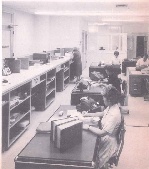
The new sleek and time saving general office of the smart new City Hall reconstructed from the Old Courthouse.
