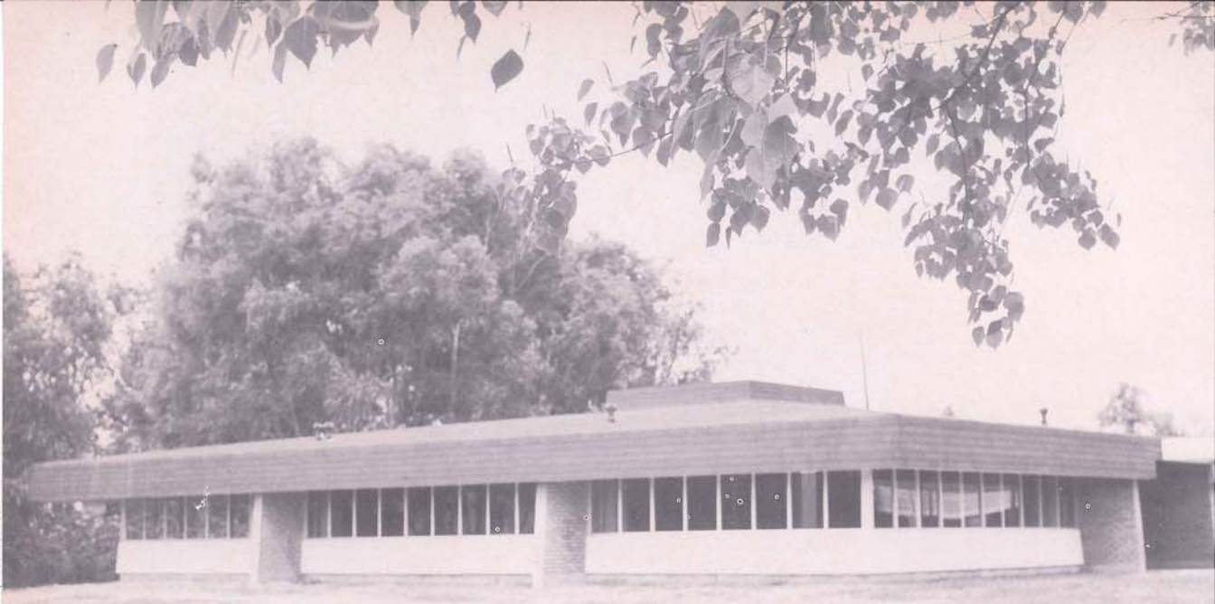
Exterior view of new classrooms at Lake Side School for Exceptional Children. Mrs. Dorcas Peters is Principal.
