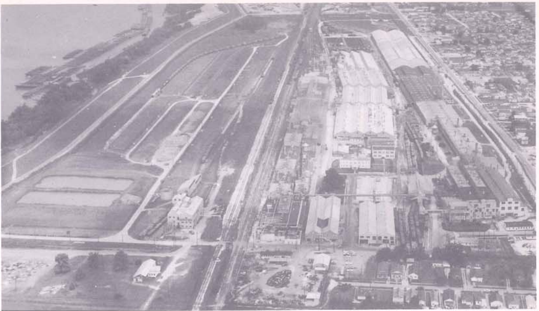
At this Celotex plant at Marrero in Jefferson Parish, the largest plant of its kind in the world, 250,000 tons of bagasse annually are processed into a production of over 1300 items. This 150 acre plant is served by 10 miles of railroad track, a fire department, ambulance facilities and a medical staff. Bagasse is the waste material of sugar cane after the juice has been squeezed out.
