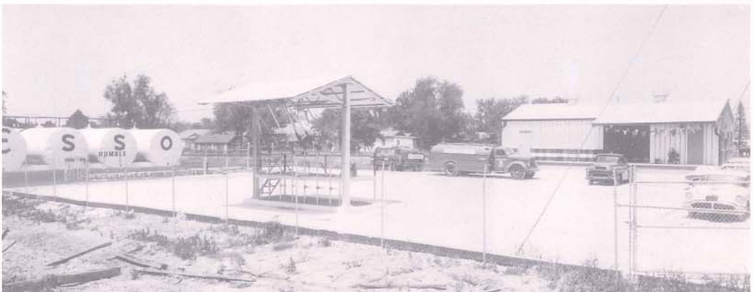
Pictured above is the Hecker Oil Company—distributing Humble Oil and Refinery products and serving Jefferson's East Bank.
