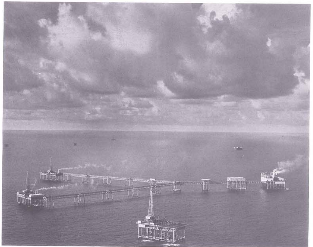
Freeport Sulphur Company's man-made steel island off-shore mine is shown in this pre-hurricane aerial view. Although heavily damaged when the eye of Hurricane Betsy passed over it, the $35 million structure off Grand Isle was quickly repaired and put back into production.
