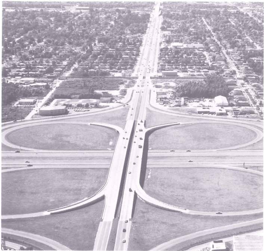
Hub of East Jefferson's major streets system is Causeway Blvd.—Interstate 10 cloverleaf. Scheduled for opening this year is extension of I-10 to Veterans Hwy. completing a 12 mile high speed, limited access expressway connecting Kenner and New Orleans.
