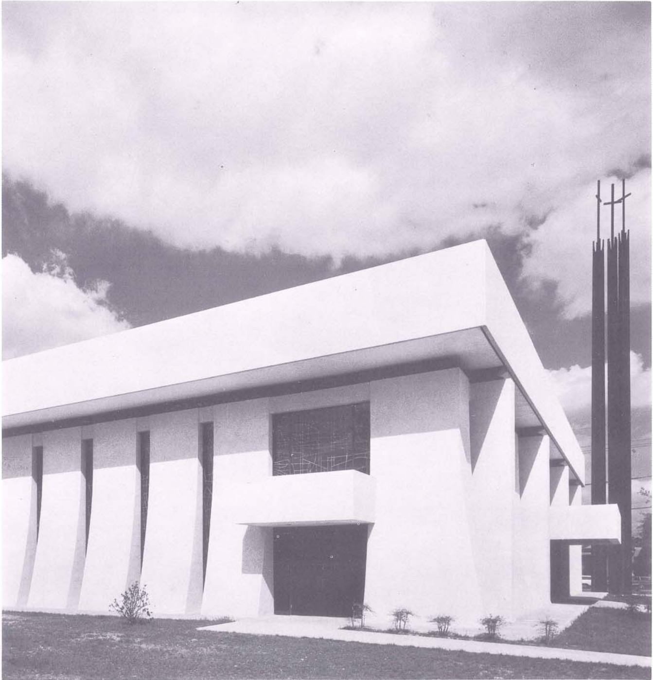
Award-winning $350,000 St. Anthony Catholic Church in Gretna replaces a 47 year wooden structure. The 97-foot steel crosses stand at the corner of Franklin and Burmaster. Finished in textured concrete, the 700 seat church is 100 by 110 feet, 28 feet high and free of interior columns.
