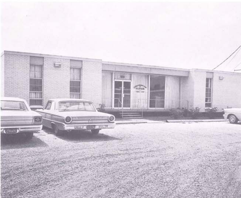
Kenner's modern Sewerage Treatment Plant No. 1 opened April 8, 1965 at 1901 24th St. just off Williams Blvd. Construction on a second plant to serve District No. 2 will begin in 1968.
