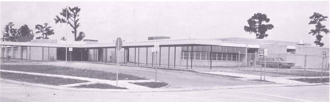
The New Catherine Strehle elementary school in Avondale
