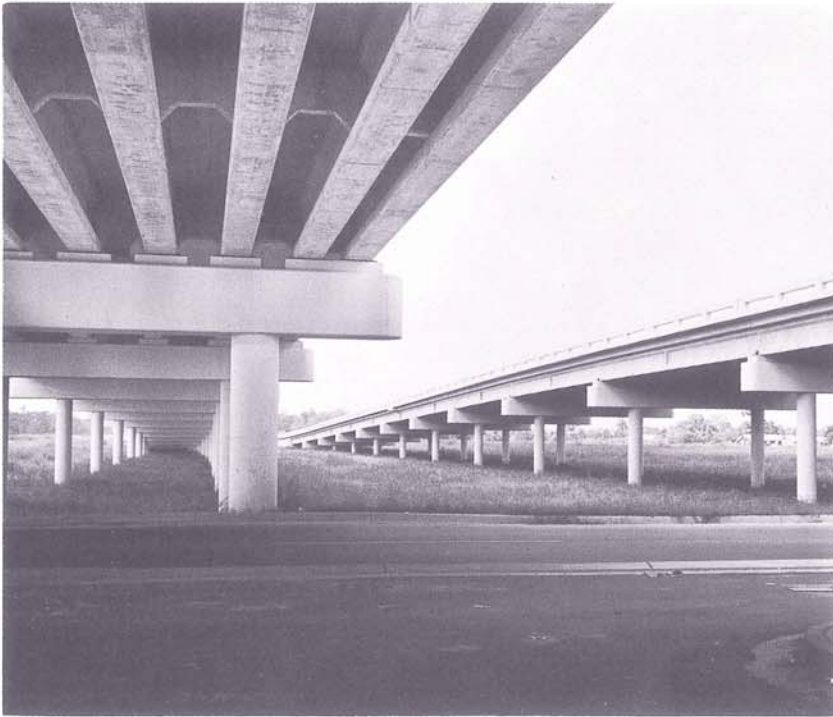
Interstate highway 10 overpass at Williams Blvd. in Kenner is shown here.
