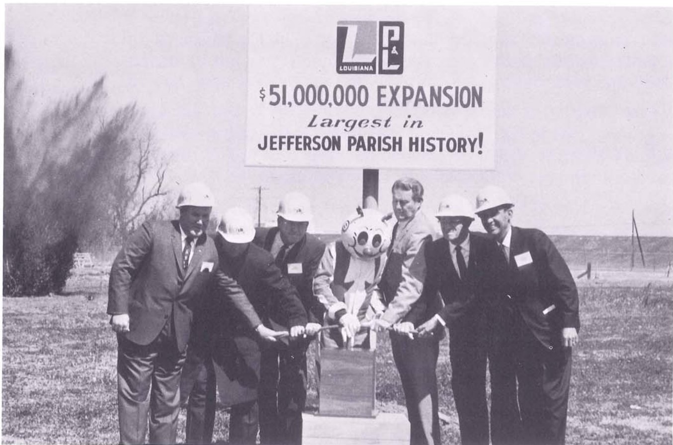
Reddy Kilowatt, joined by LP&L and Jefferson Parish officials, sets off a dynamite charge initiating construction of LP&L's $51-million expansion project at Ninemile Point steam-electric generating station near Westwego. Pictured from left to right are: Charles M. Miller and Harold L. Molaison, Jefferson Parish Councilmen; Tom F. Donelon, Parish President; Reddy Kilowatt; Nat B. Knight, Louisiana Public Service Commissioner; G. C. Rawls, LP&L Chairman of the Board; and Ernest J. Tassin, Mayor of Westwego.
